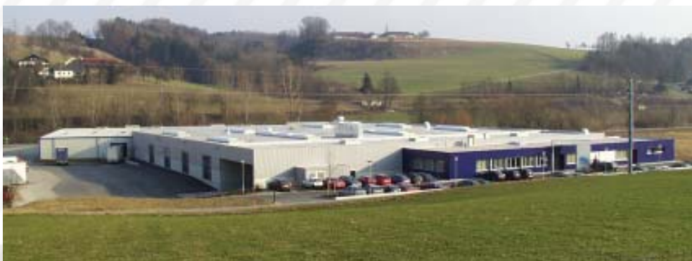
The new built plant of Eurofoam / pactec in Kremsmünster.
