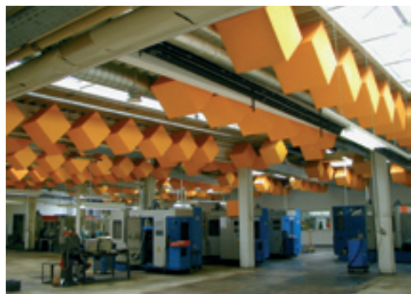
Audiotec absorbers are excellently suited to improving acoustics and reducing noise levels in manufacturing and multi-purpose halls. They are moreover individually shape-able.
